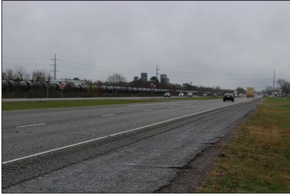
Photo 1 – Looking northeast along US 90 near the southwest project limit.
