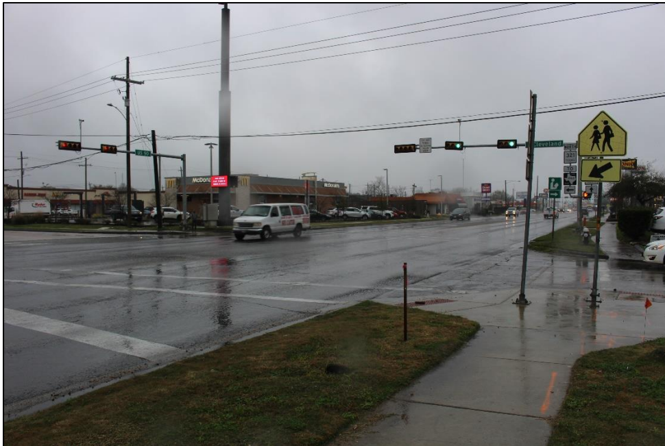
Photo 20 – Looking northeast at the US 90 and N. Cleveland St. intersection.
