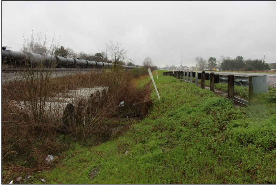
Photo 23 – Looking northeast at culverts along the north shoulder of US 90.
