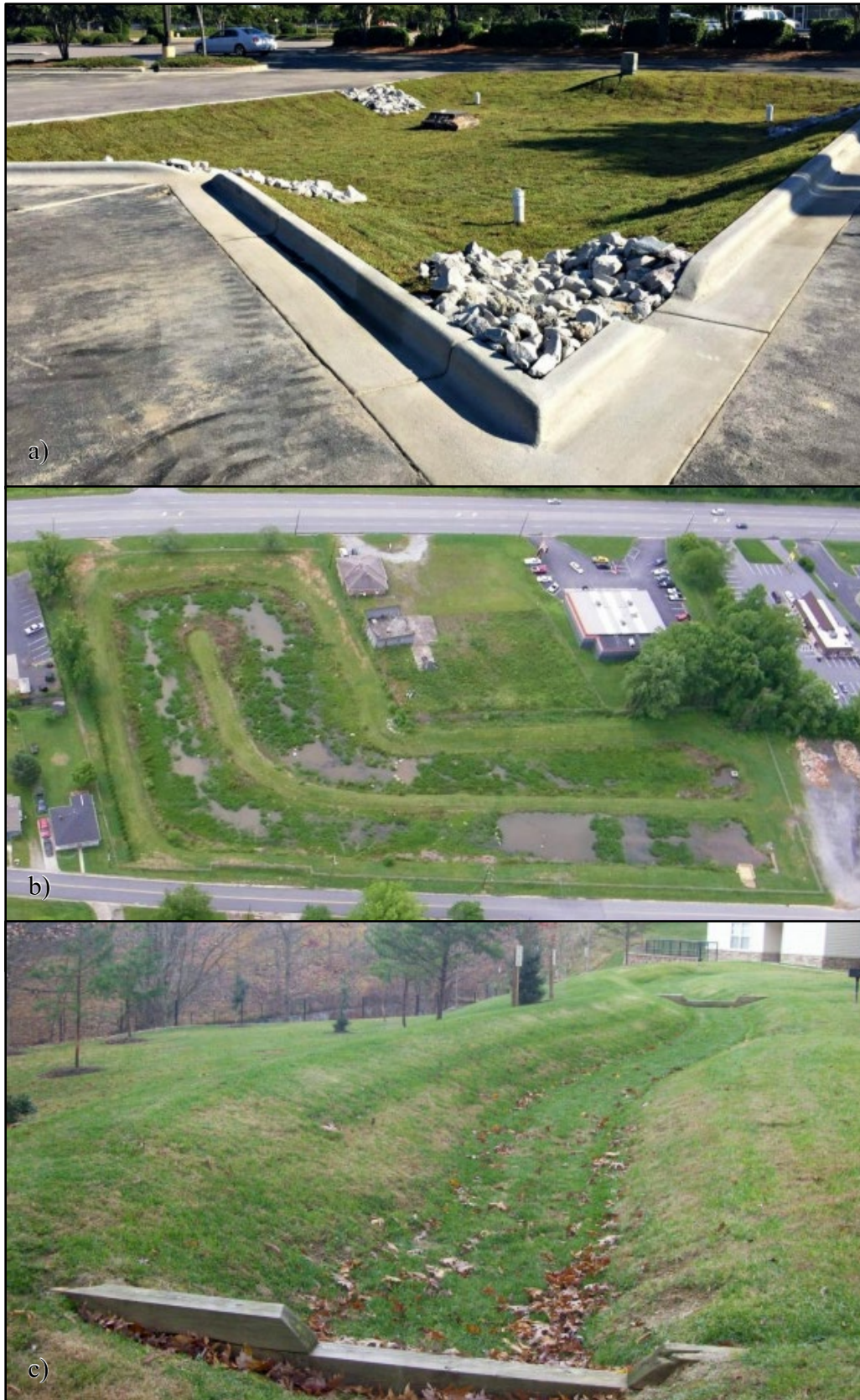
Figure 2 - Common SCMs. From top to bottom: a) a bioretention cell, b) a stormwater wetland, and c) a treatment swale. Images source: Stormwater Design Manual, NCDEQ, 2020.
